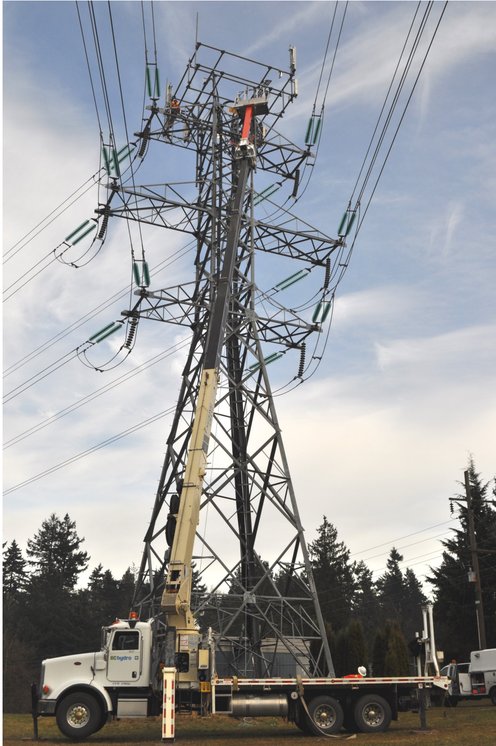
765kV AC/500kV DC Insulated Work Platform with Hydraulic Articulation
